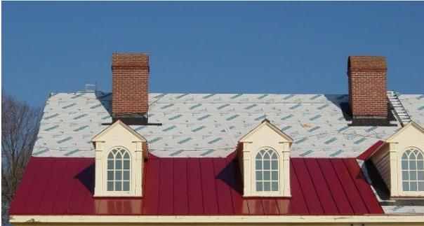
**If replacement is necessary use a metal seam roof similar in dimensions, spacing and crimping as the original.**
