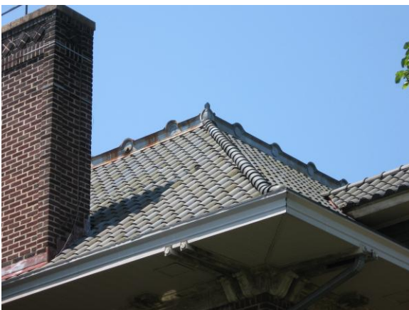
Original clay tile roof at 2701 Rivermont Avenue.
