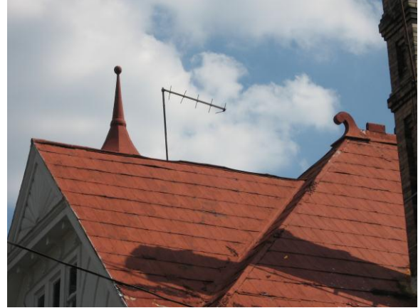
Original metal shingle roof at 429 Rivermont Avenue.
